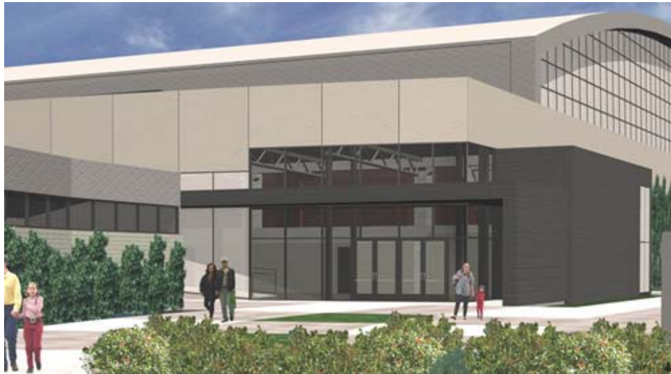
Figure 3 – View of Main Entrance of Natatorium (showing precast concrete panels, metal wall panels, and glazed curtain walls)
